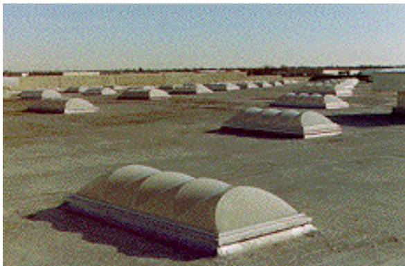
Figure 8: Compound parabolic skylight
